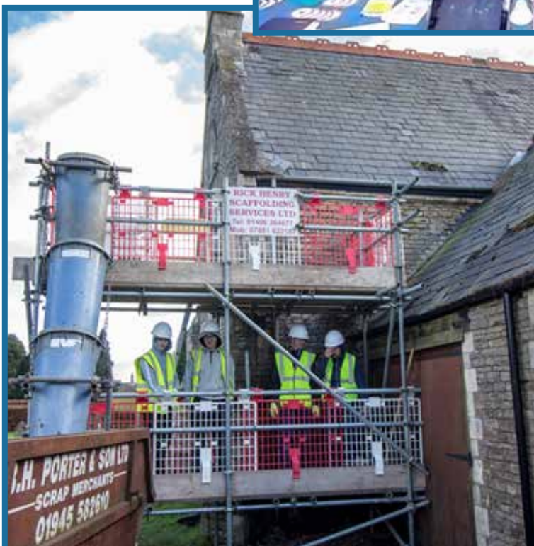
Bricklaying students from the College of West Anglia – one part of the Wisbech 2020 Vision project
